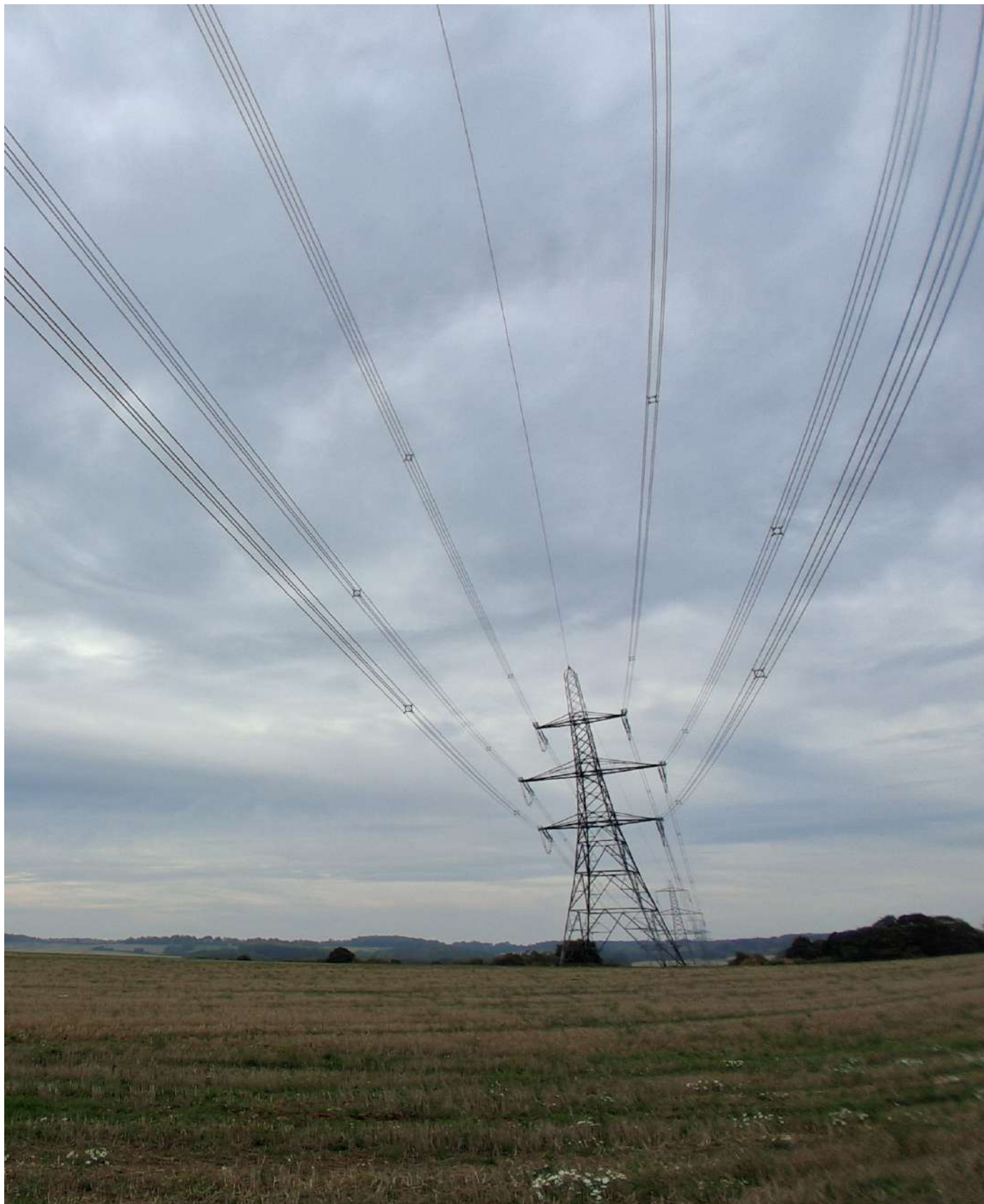
Figure 3: View to the southwest in western site parcel
