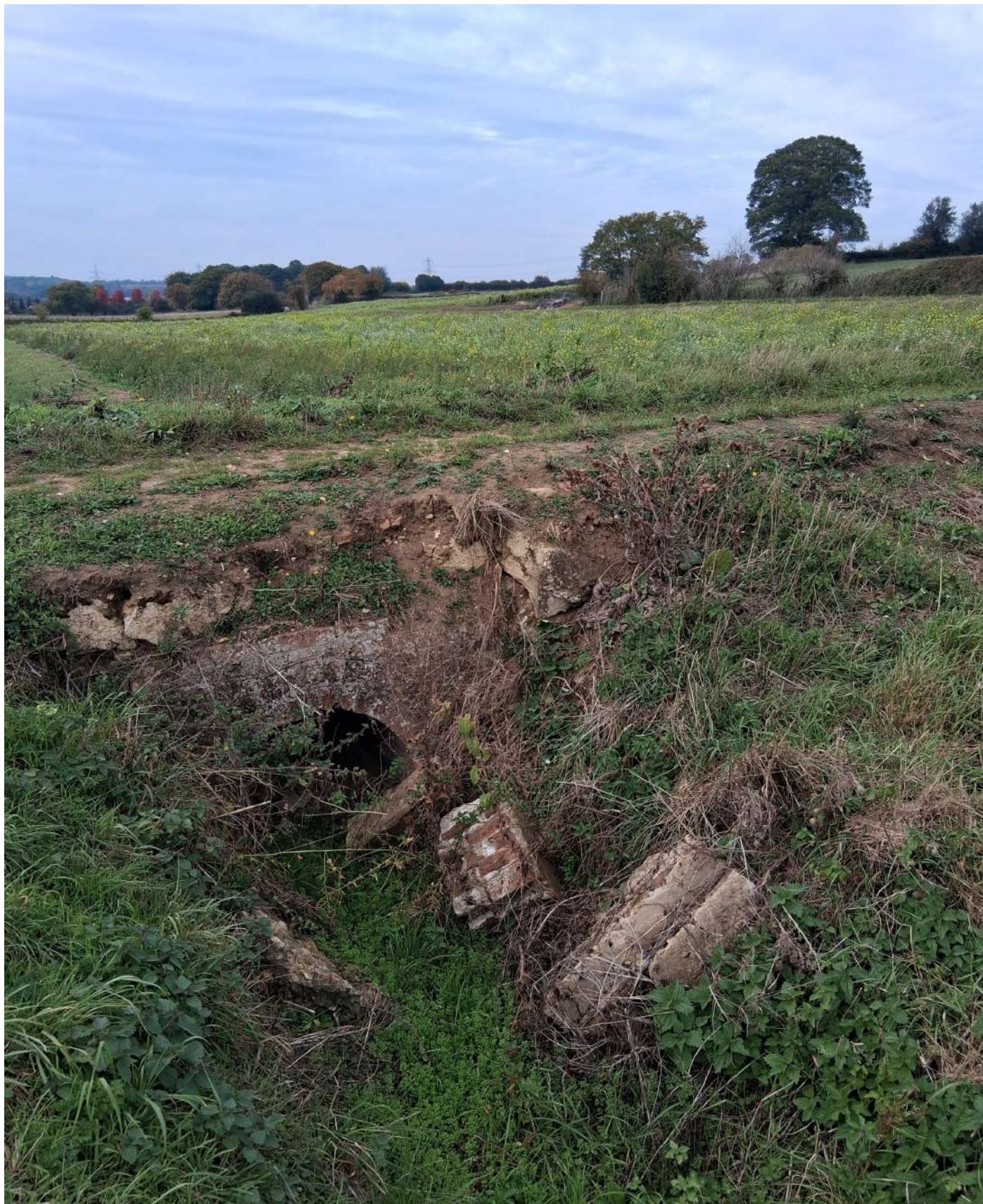
Figure 8: View of drainage ditch between central and southern site parcels
