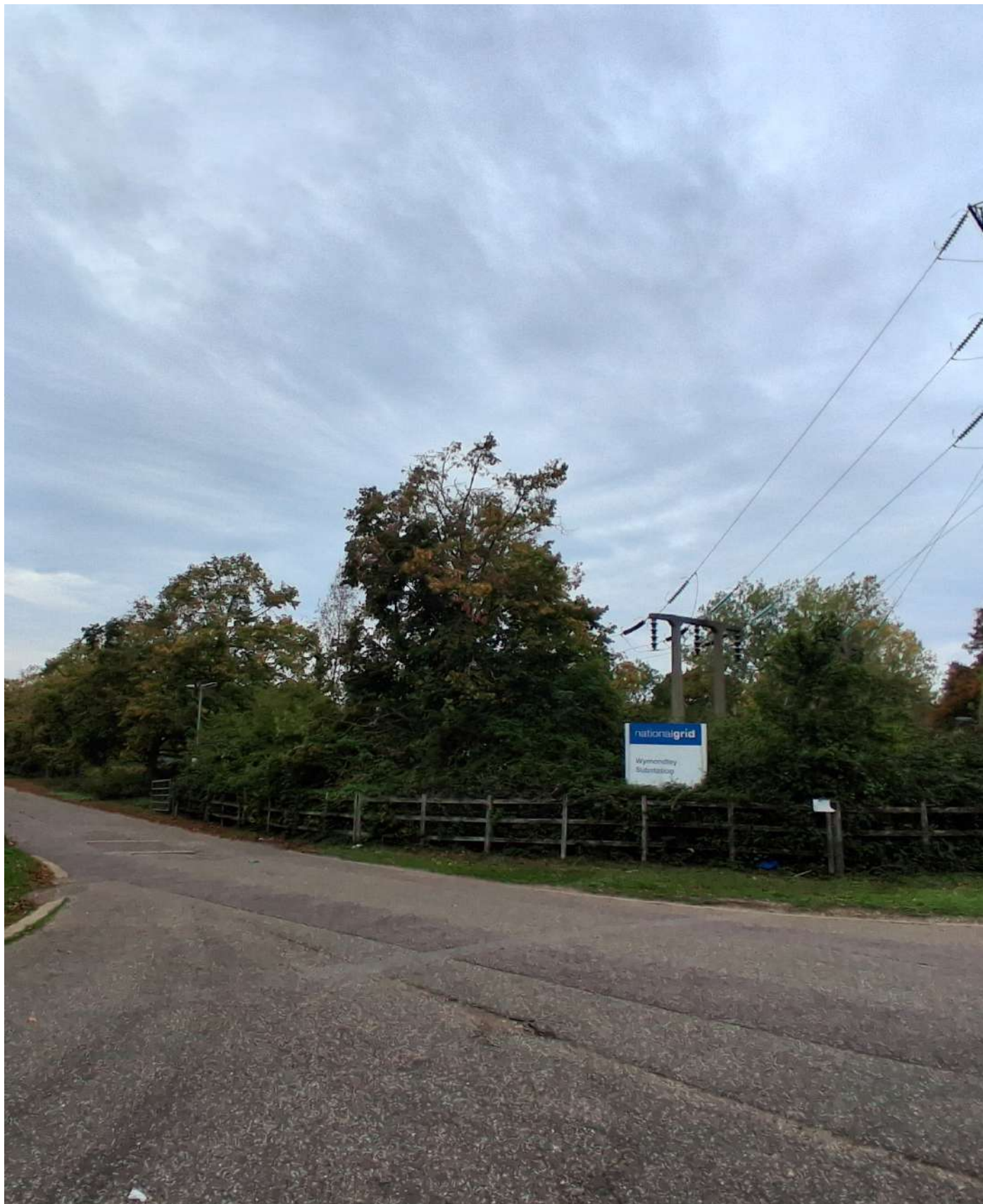
Figure 17: View of National Grid Wymondley Transformer Substation north of the site
