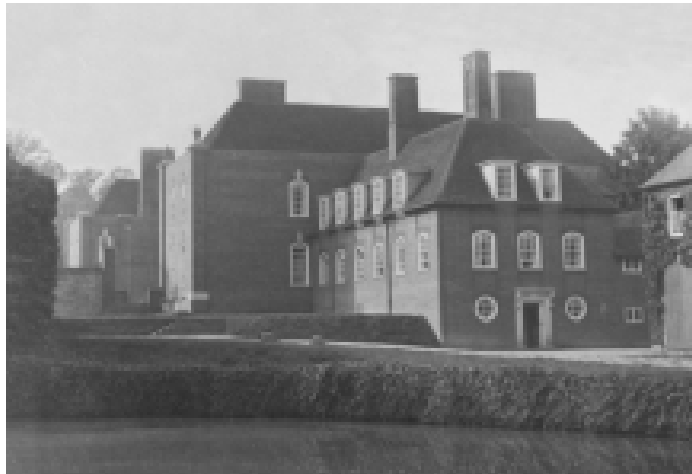
Post 1912 photo showing Lutyens' East Wing and Annexe completed prior to the 1913-14 linking section also carried out by Lutyens'.
