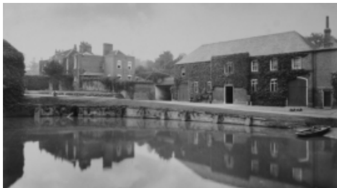
Pre- 1909 photo showing the East End of the building prior to the Lutyens' East Wing.
