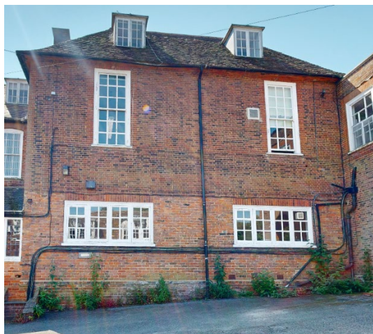
Stable Block North Elevation - First Floor tall sash windows are later C20 additions.
