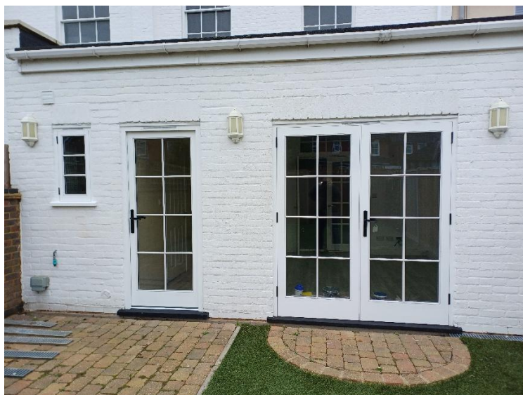
New timber window & doors installed. Brickwork painted white to match host building
