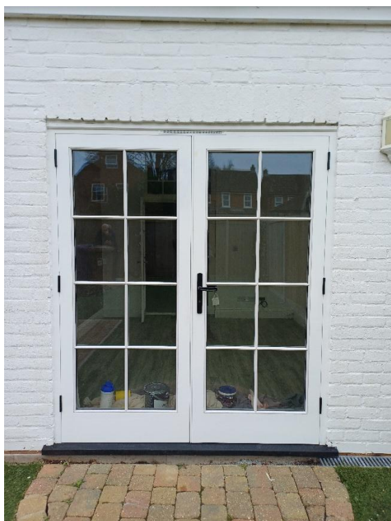
New timber double doors to playroom from garden
