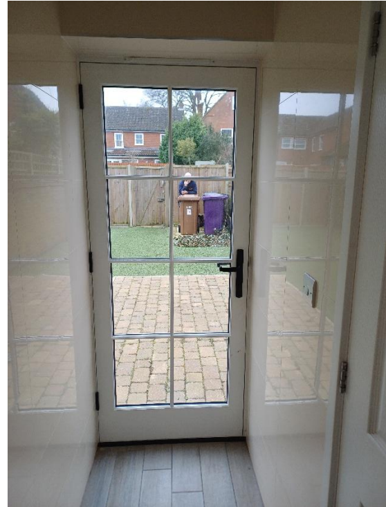
New timber rear door
