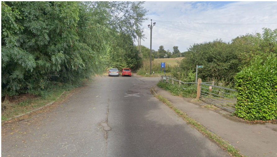
Existing cul-de-sac off Stevenage Road and only access to proposal
