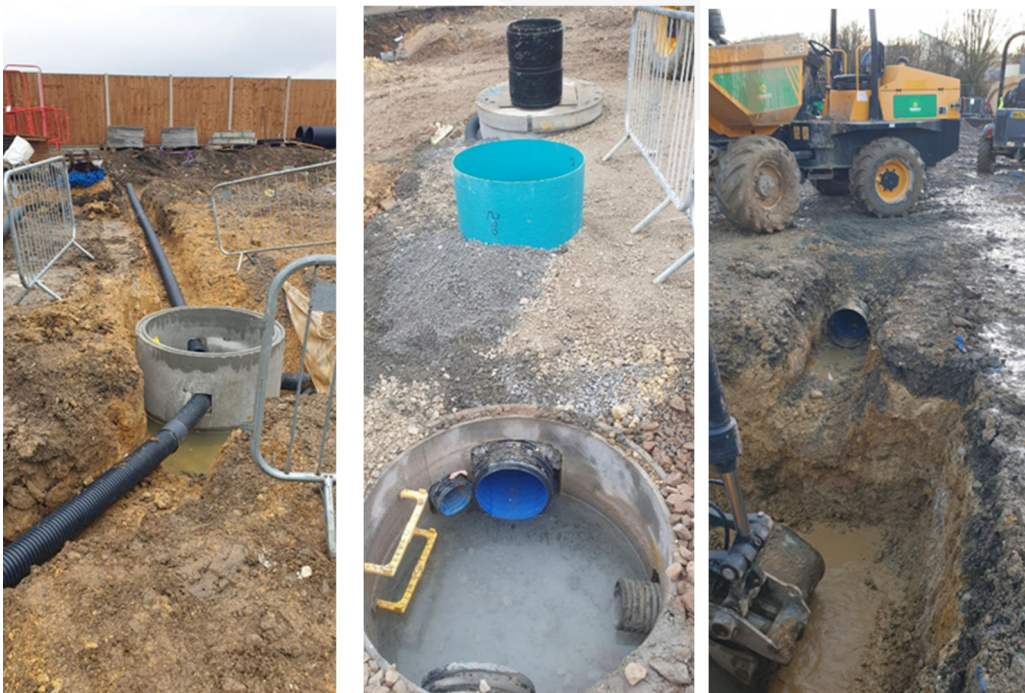
Figure 4: Piped network during installation
