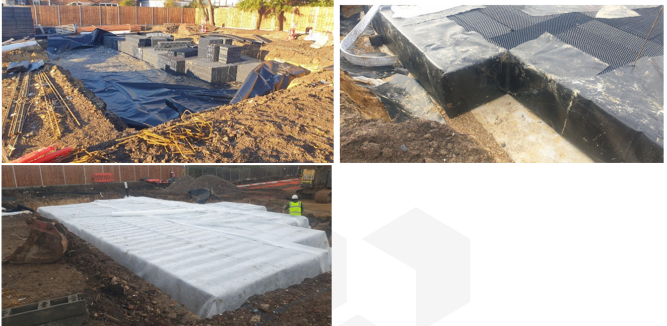
Figure 3: Geocellular crate attenuation being installed with impermeable liner and protective fleece
