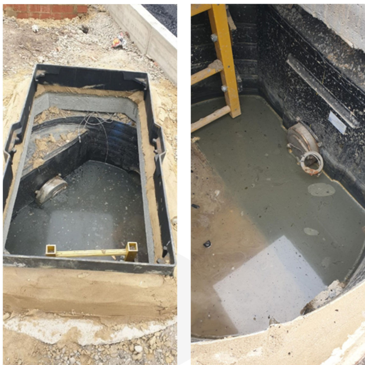
Figure 5: Crown vortex flow controls in-situ. Final site control on left and intermediate control on right.
