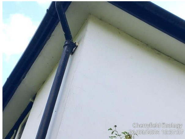
Figure 10: Example of the tight soffit box
