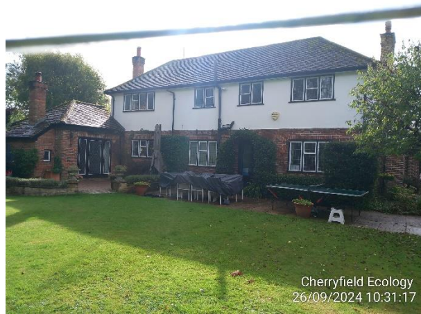
Figure 3: Example of B1's exterior
