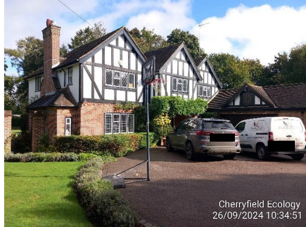
Figure 2: Example of B1's exterior
