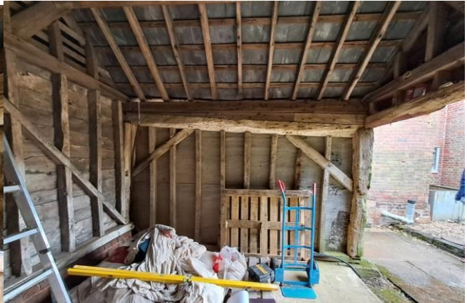
Internal front wall
