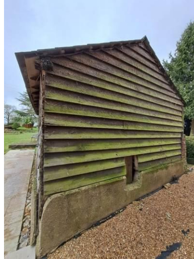
Henhouse external RHS
