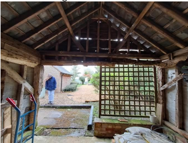
Internal Existing Entrance
