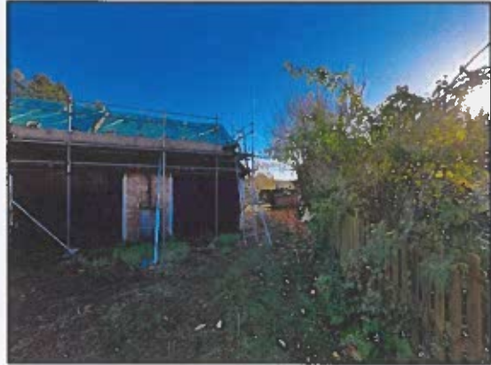
Fig 5 – Front elevation and adjacent neighbour's garden.
