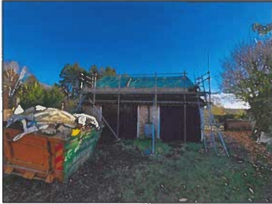
Fig 4 – Front elevation of the existing out-building.
