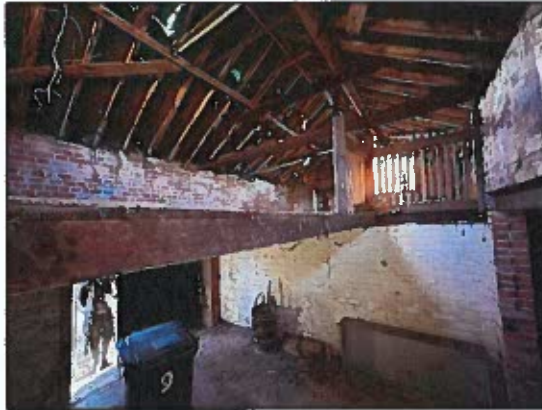
Fig 12 – General internal view looking north.
