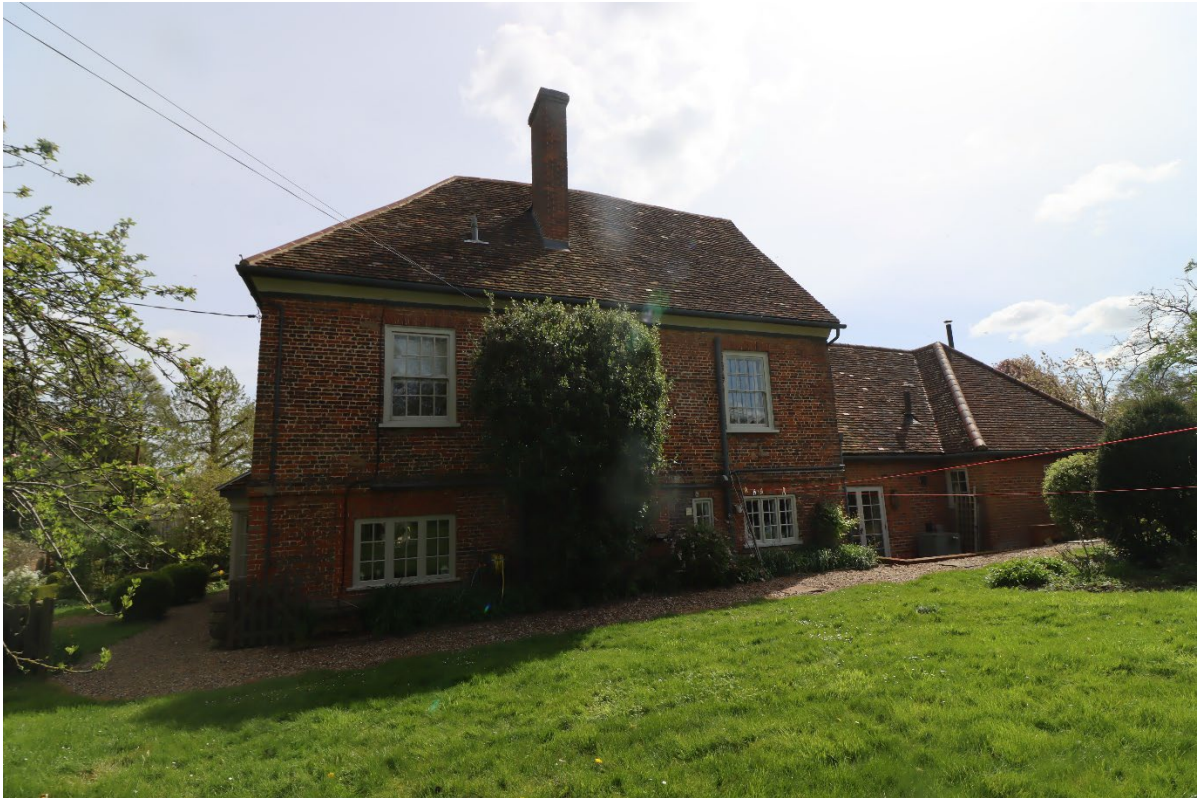
Image 11: Church Farm House side elevation (west facing)
