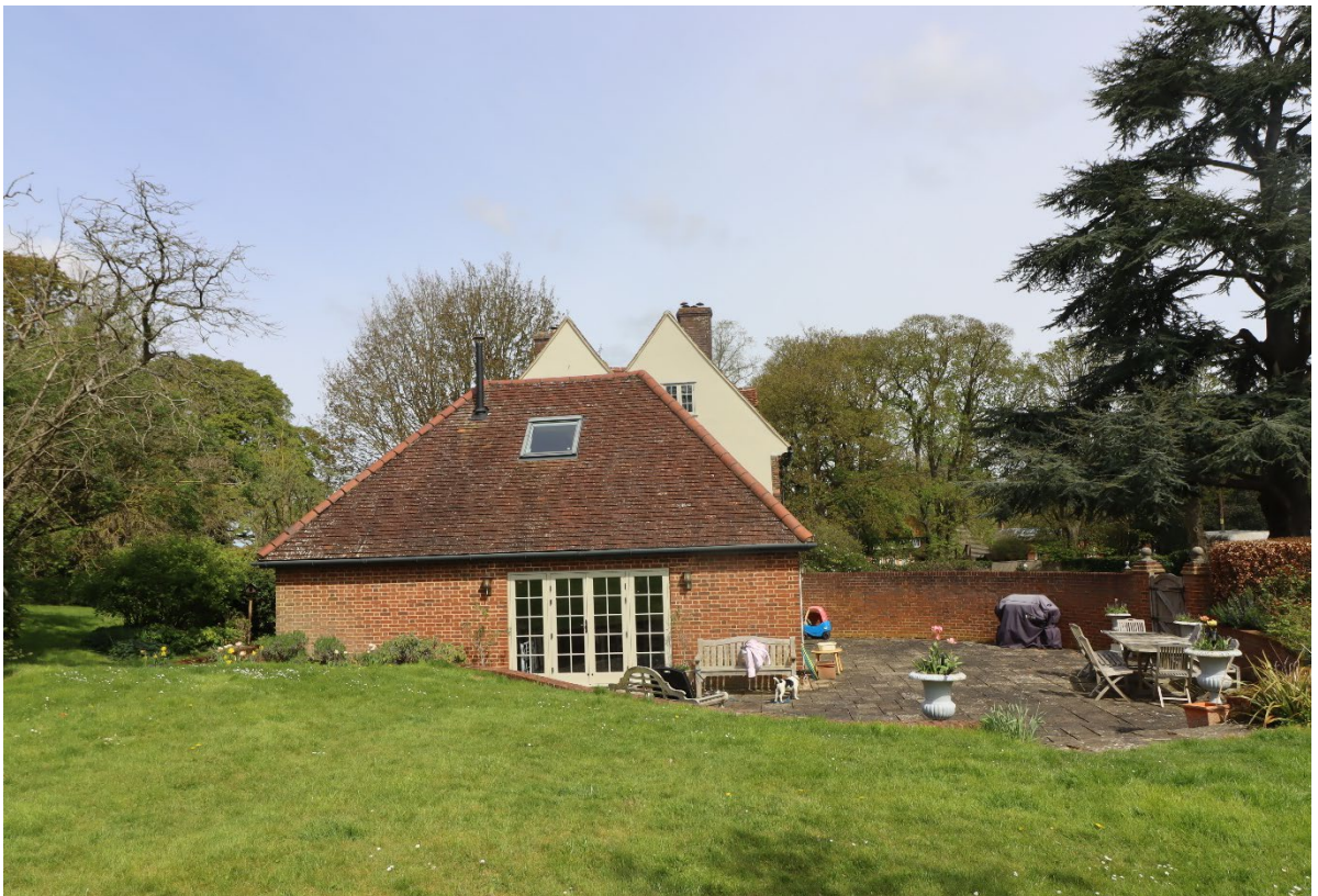
Image 12: Church Farm House rear elevation (south facing)
