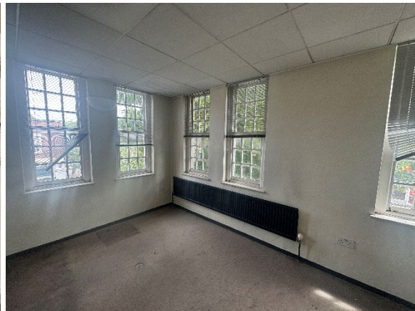
Internal view at first floor level
