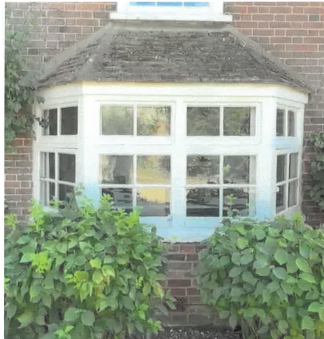
Photo of existing bay window
