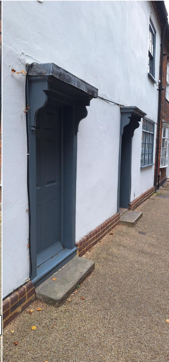
Examples of existing doors to Church Street
