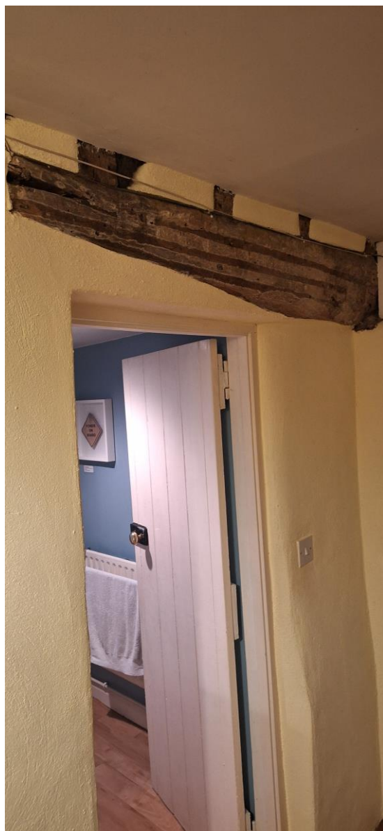
Internal door to WC - to house
