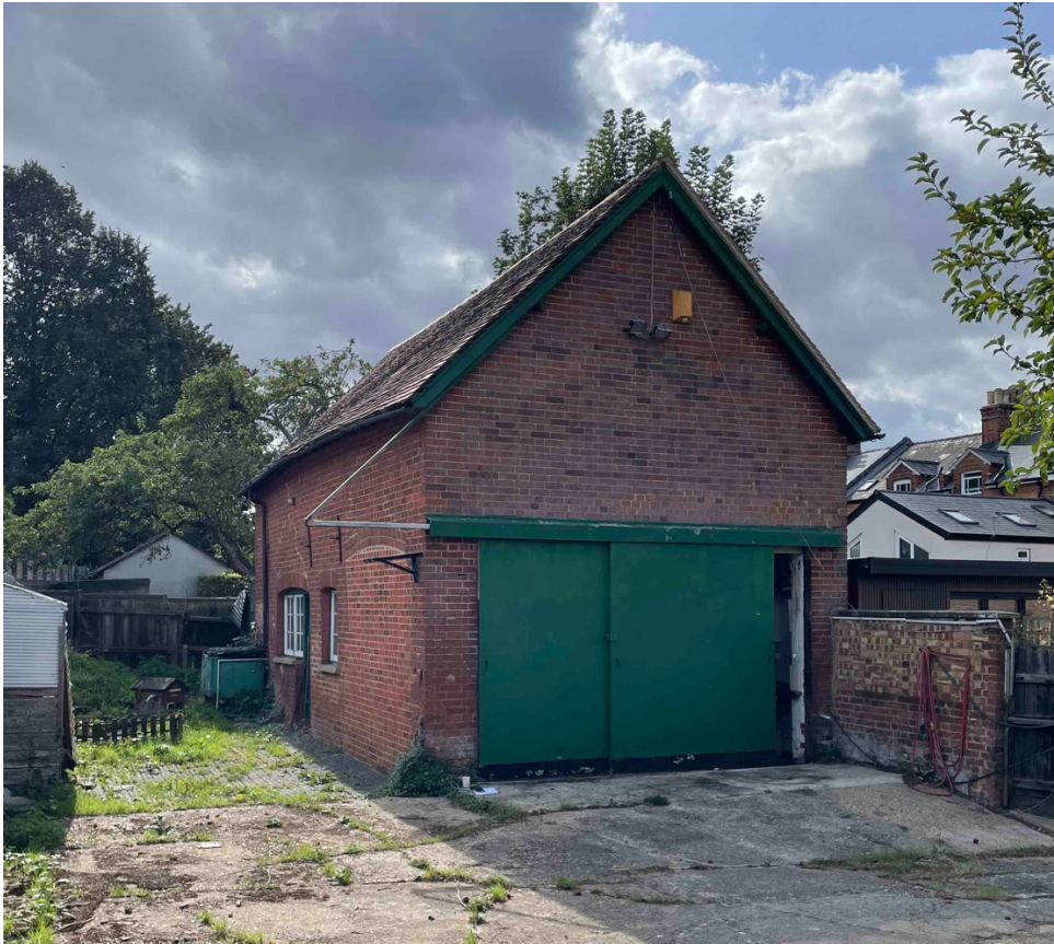
Existing Brick Barn
