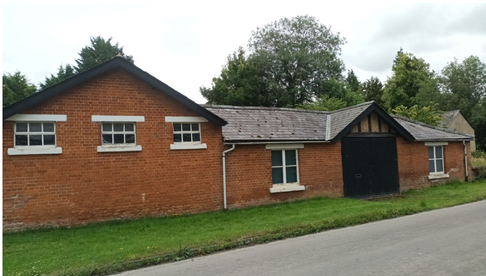
Photo 1: View to the east showing the barn in the west of the site
