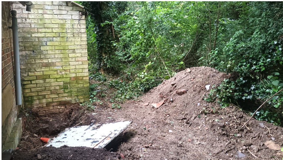
Photo 8: View to the north showing the location of TP04
