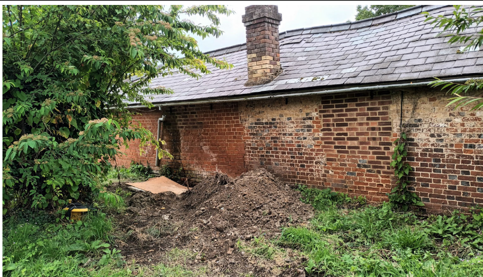
Photo 2: View to the northwest showing TP03 in the south of the site
