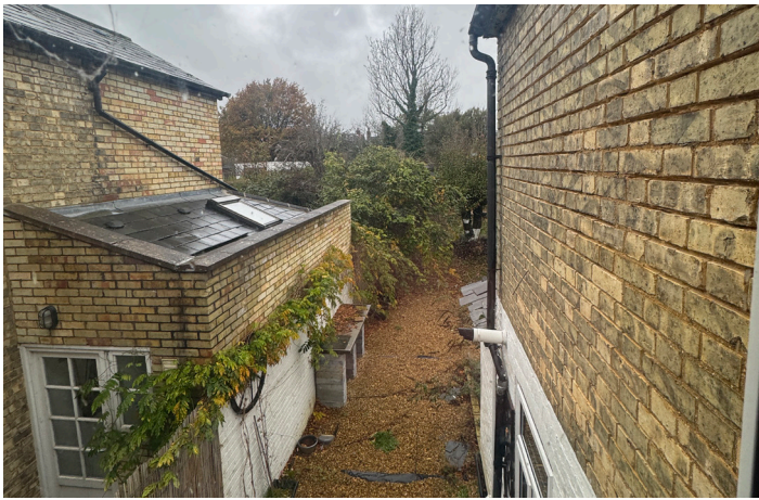
Side/rear extension at No.50 (with rooflight)
