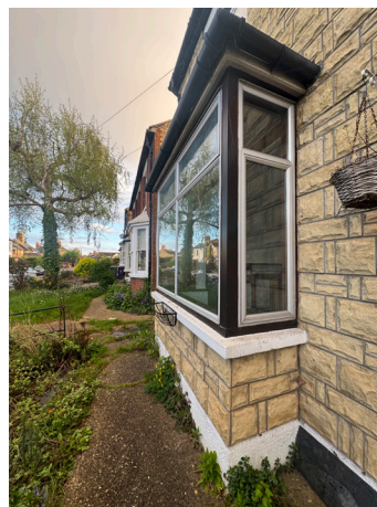
Stone cladding to the front elevation
