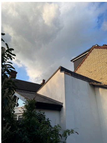
Stepped roof profile of No.52s' single-storey extension
