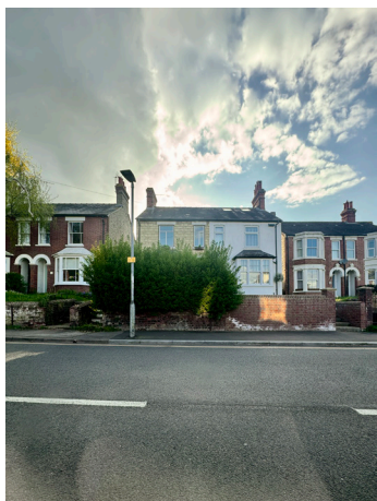
2 No. rooflights can be seen within the slate-covered roof of No.52
