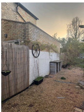
Side-rear extension of No.50- height 3m at boundary (date unknown)
