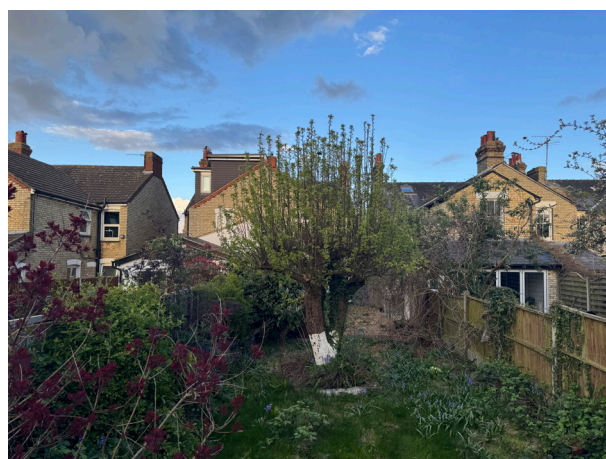
Rear view of Nos. 50-53 including L-shaped rear dormer at adjoining neighbour of No.53
