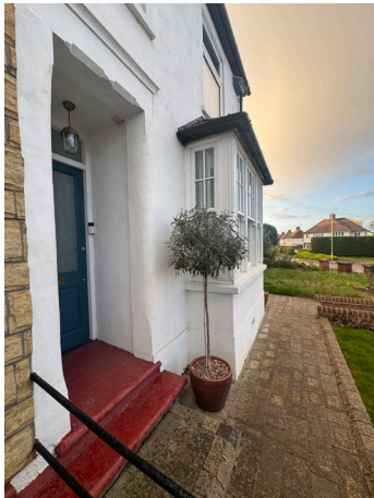
Adjoining No.52 with clean, white render finish and double-glazing
