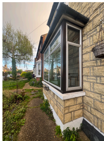
Stone cladding to the front elevation
