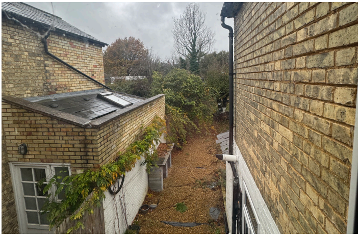
Side/rear extension at No.50 (with rooflight)
