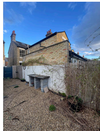
Rear view of No.50s' side/rear extension (date unknown)
