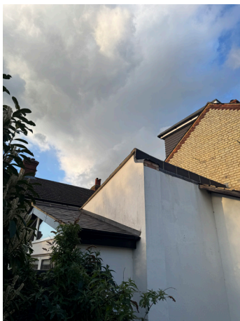
Stepped roof profile of No.52s' single-storey extension
