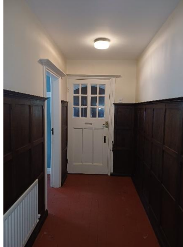
Original front entrance door
