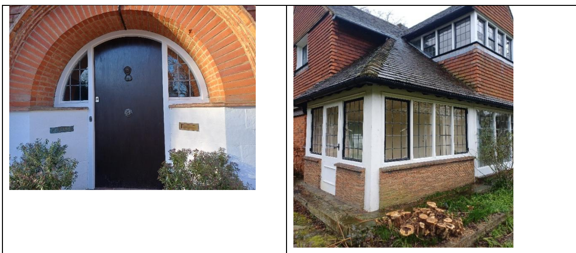
1. Door installed in front of original entrance to be removed
