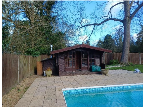
Old swimming pool outbuilding
