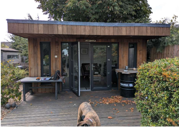
Existing Garden Room
