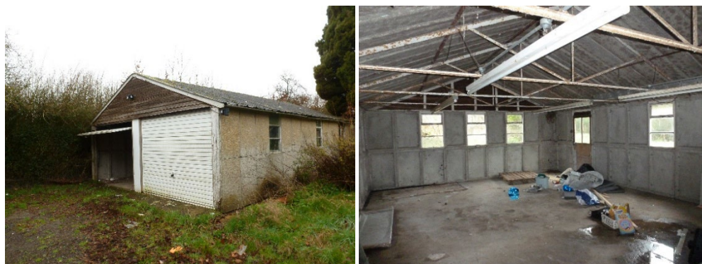
Plates 5 & 6: Photographs of the exterior & interior of the detached garage
