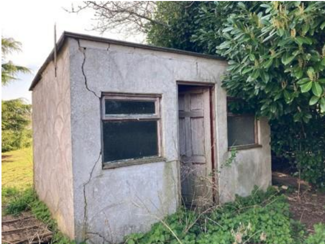
Plate 10: Exterior of outbuilding (B5)
