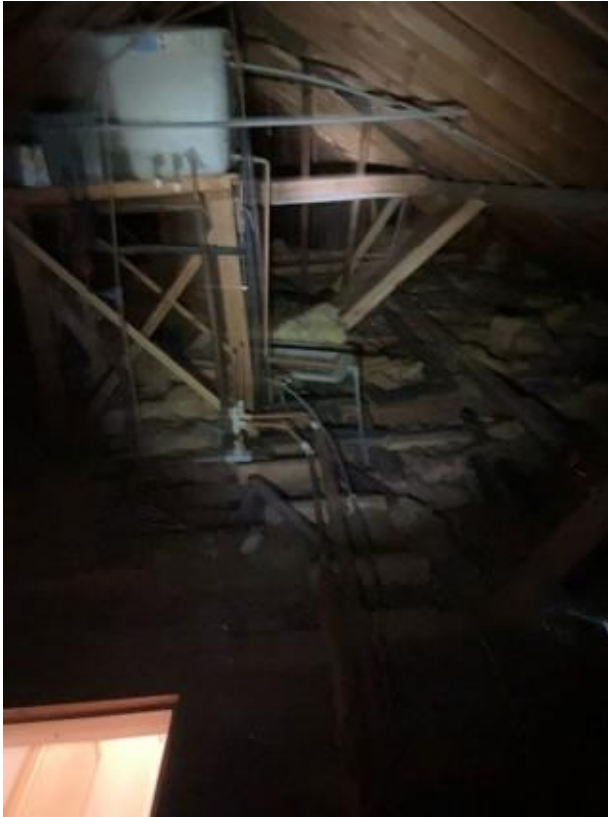
Plate 12: Loft space in bungalow (B1)
