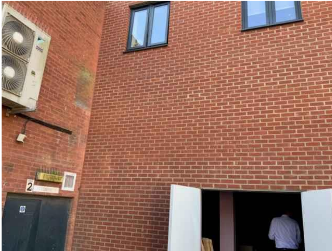
Image shows the side elevation access door which is to be bricked up
