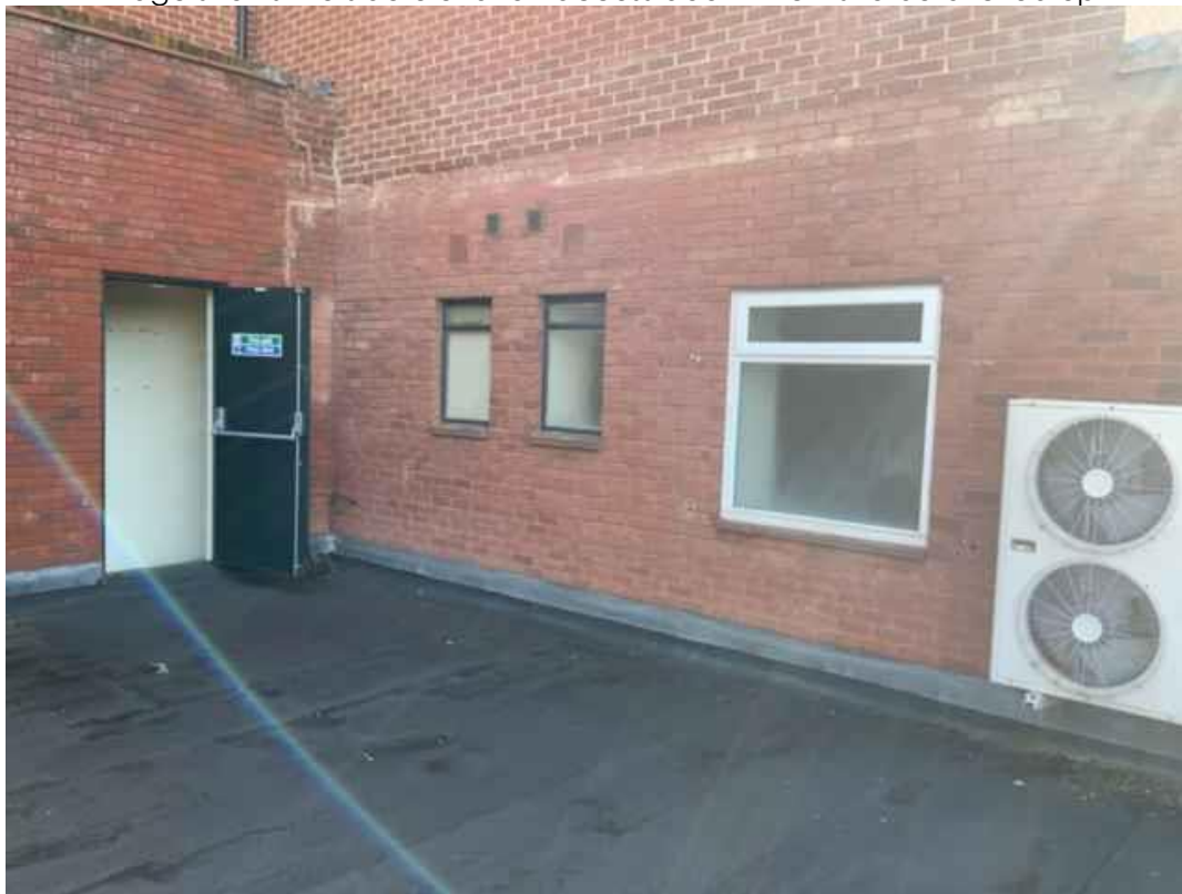
Image shows the first floor flat roof where 13 of the condensers will be installed
