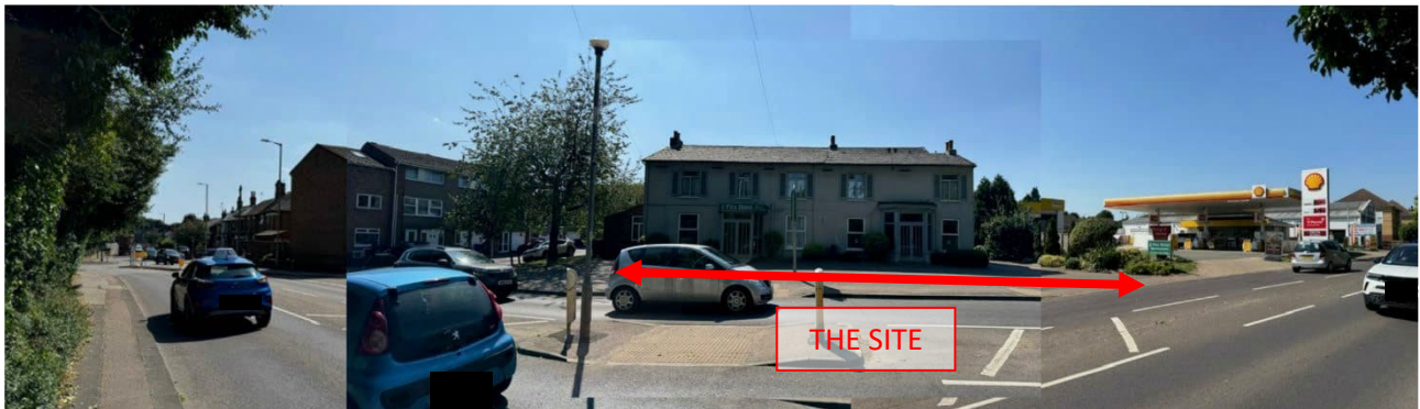
View of the site frontage looking west
