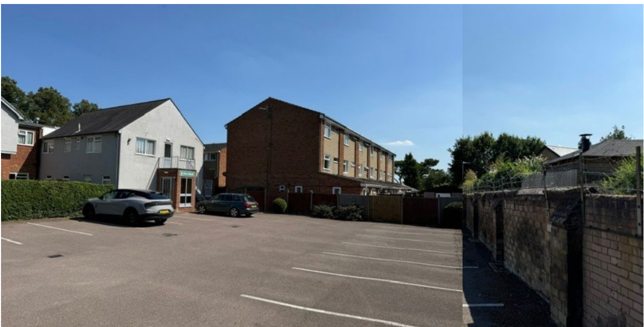
View to the south from inside rear car park of The Firs Hotel on to flank of Firs Close neighbouring buildings / gables
