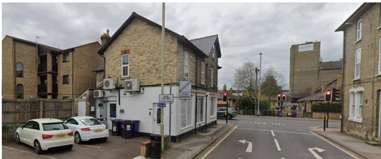
Rear and side elevation; note the three existing a/c units mounted on the rear elevation
