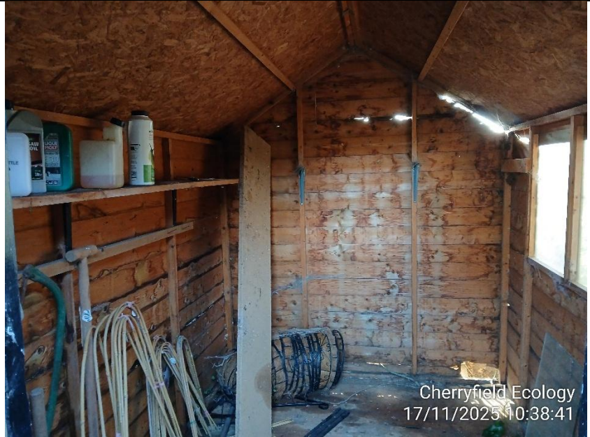
Figure 6: Interior of B2.
