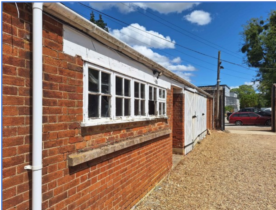
Figure 2 – View of front elevation
