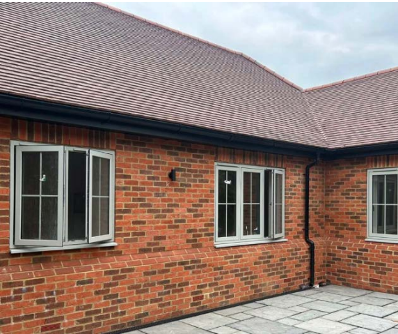
Melford Blend imperial bricks laid in an english bond to match the existing
