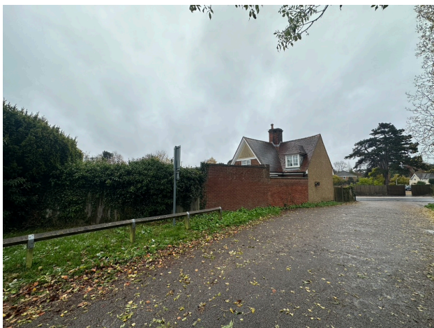
View towards Cottage from Windmill Hill
