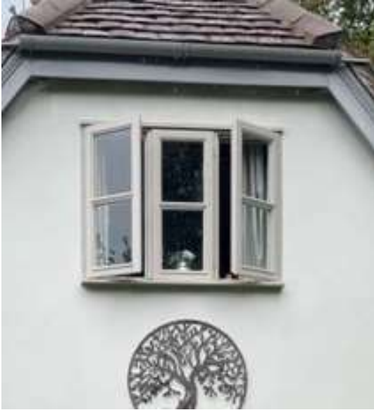
Existing timber window.
