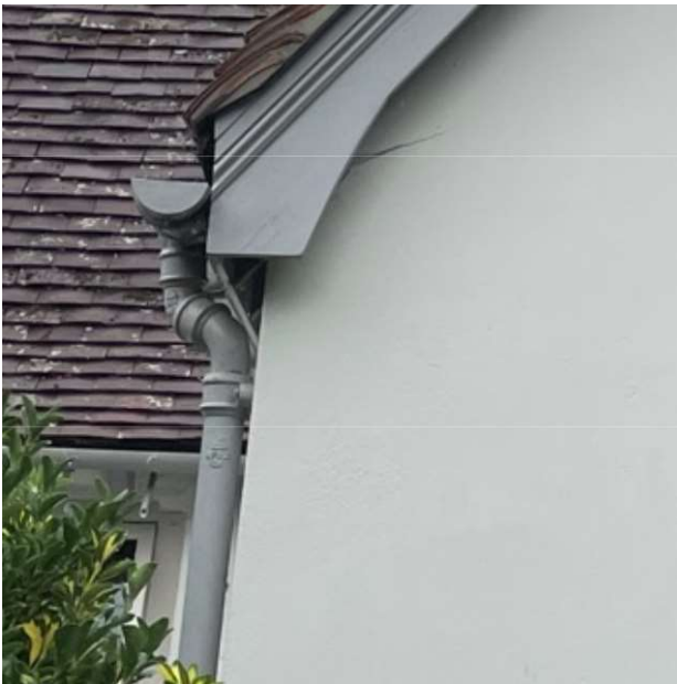
Existing gutter and downpipe
