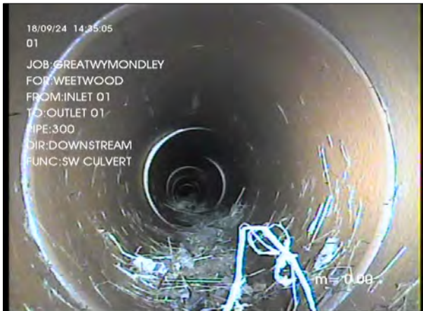
Photo: 1_2A 0m, Water level, 0% of the vertical dimension
