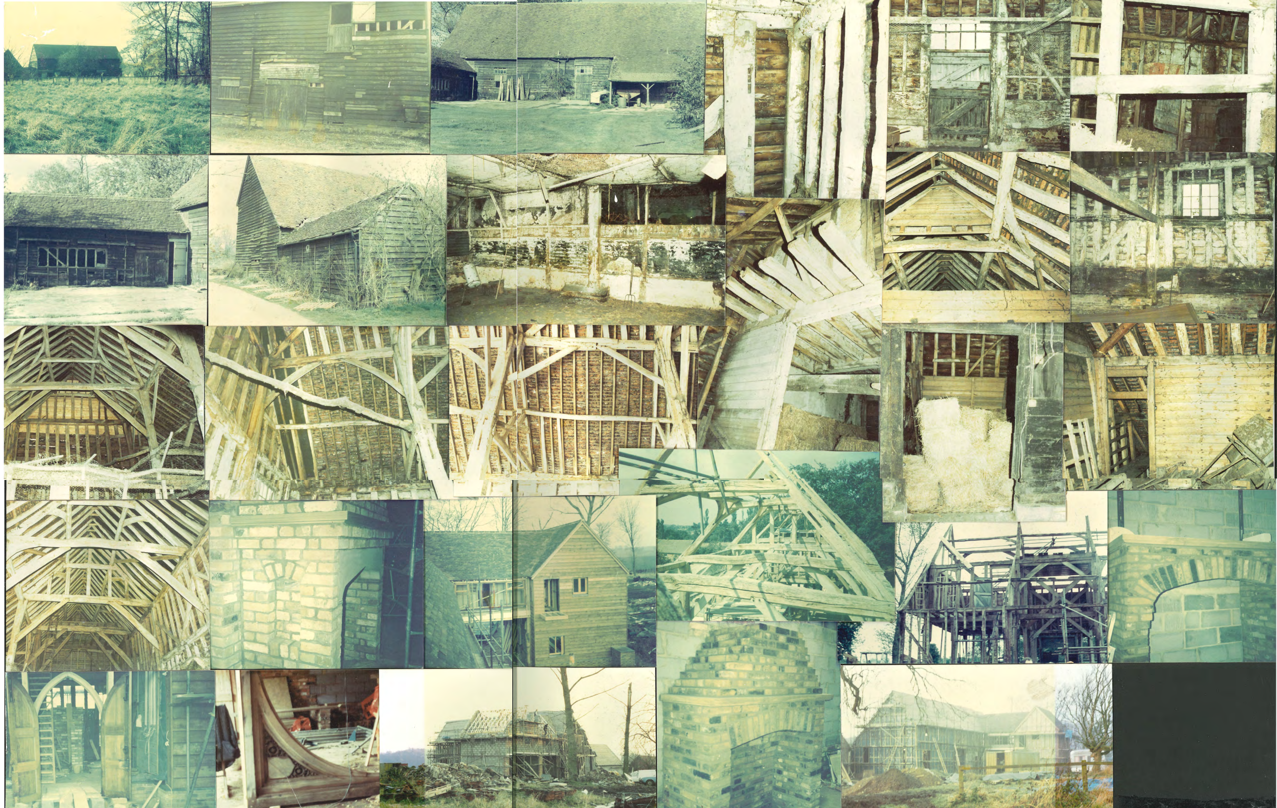
Photographs from the conversion from a barn to residential property
