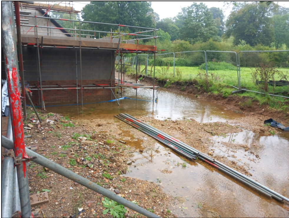
Plate 3: Southwest corner of site, facing northeast
