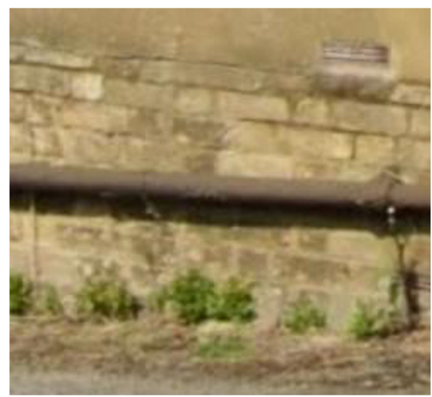
Facing Brickwork: (buff)
