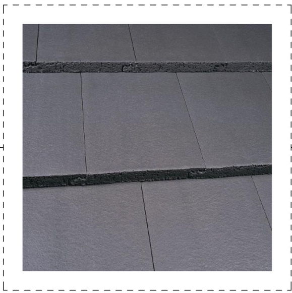
Roof Tiles: Concrete tile (grey)
