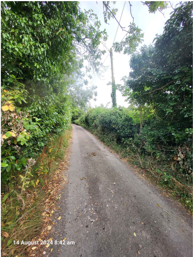
VIEW NORTH WEST TOWARDS ASHANGER LANE
