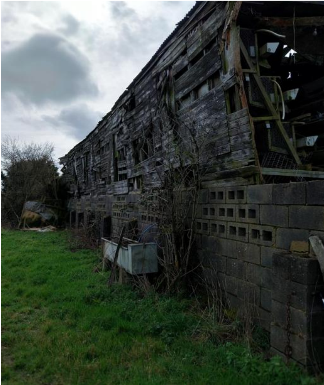
Angled view of eastern elevation
