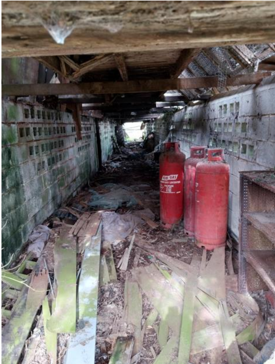
Internal photo of part of ground floor of barn
