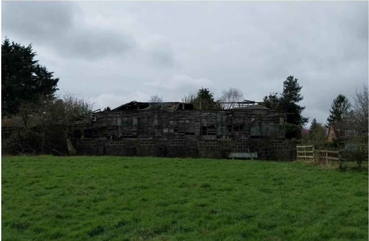
Eastern elevation of barn
