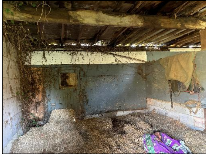
Photograph 4 Interior of stables/feed store
