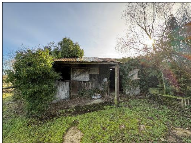
Photograph 3 Western elevation of stables/feed store
