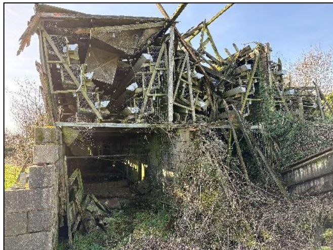
Photograph 2 Interior of chicken shed, northern elevation
