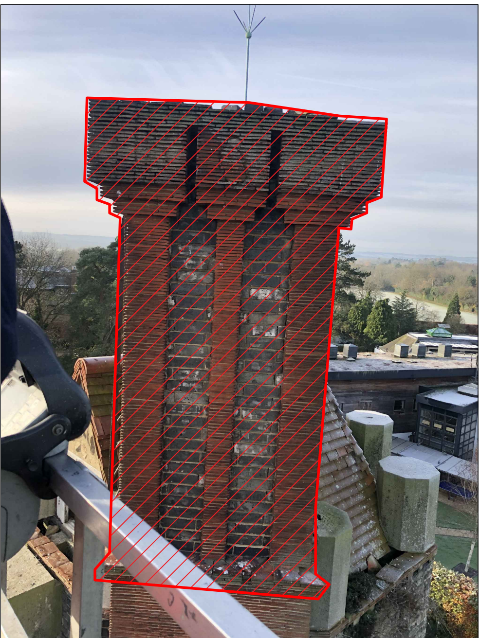
2.0 Tower - NE elevation
