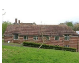
3. Science Block roof
