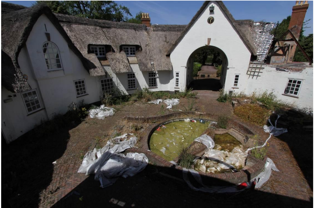
View of the existing internal courtyard
