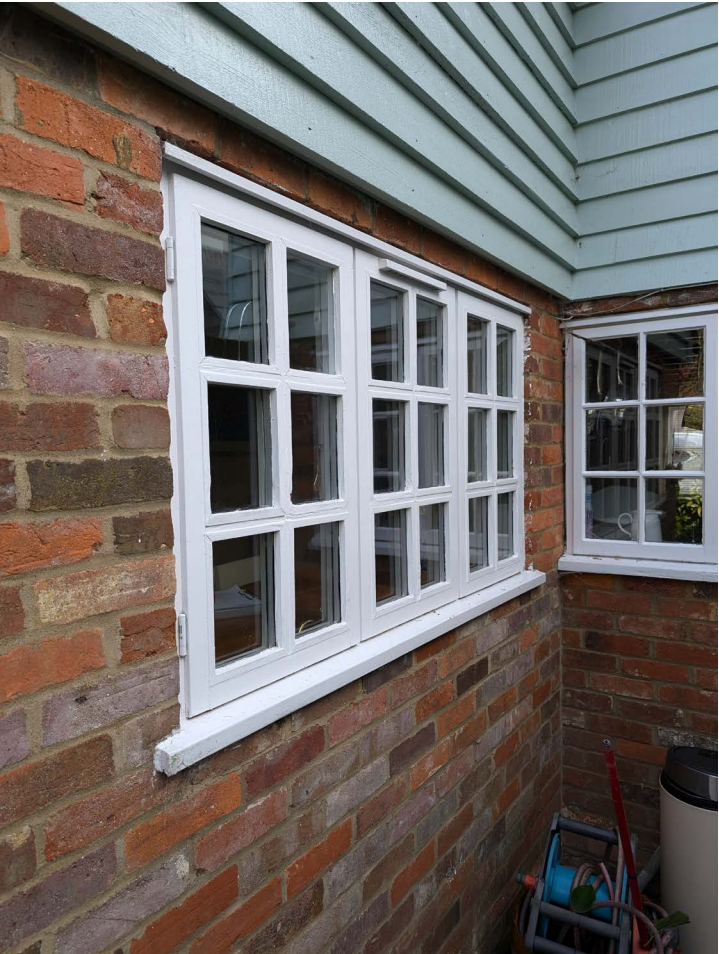
windows on newest extension
