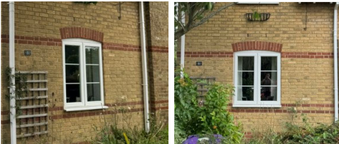
Examples of existing double-glazed uPVC casement windows + examples of the distinctive brick banding
