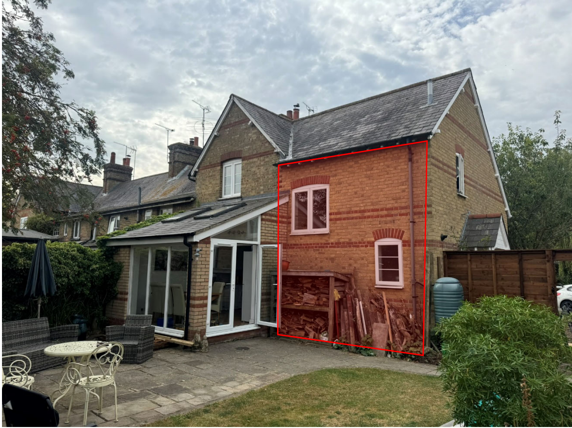
Property as seen from the rear, showing late C20 extension + later C21 single storey extension. Location of proposed extension shown in red.
