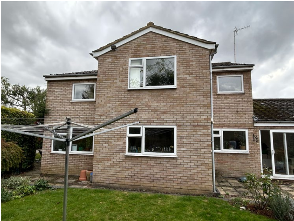
Rear Facade (North-East)
