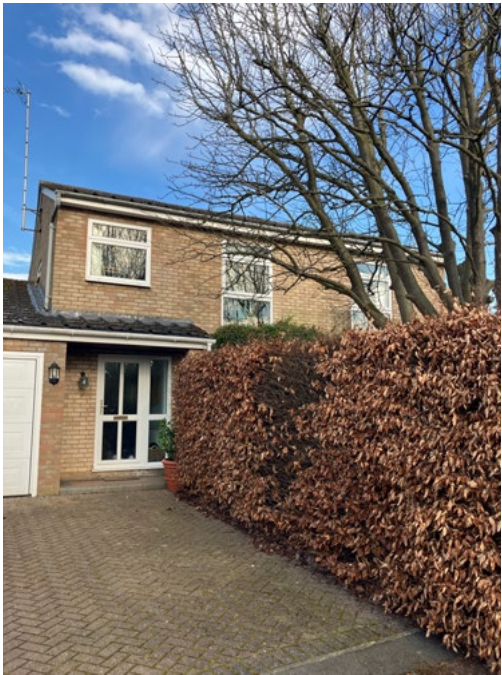
Front Facade (South-West) Approach view from driveway
