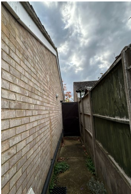
Side Facade (North-West) View from rear garden
