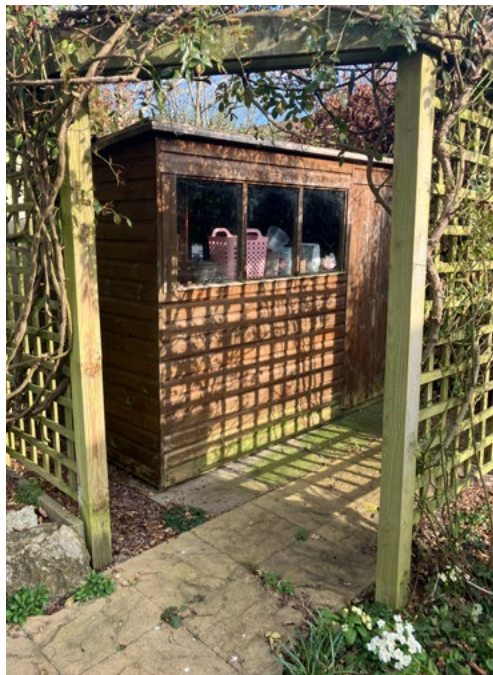
Rear garden, existing garden shed
