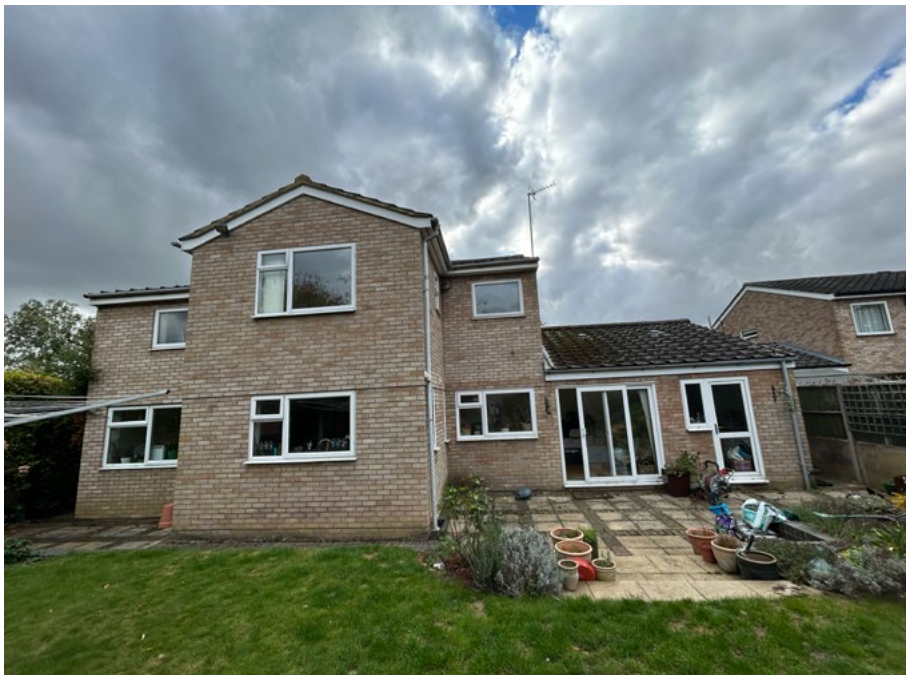
Rear Facade (North-East) View from rear garden
