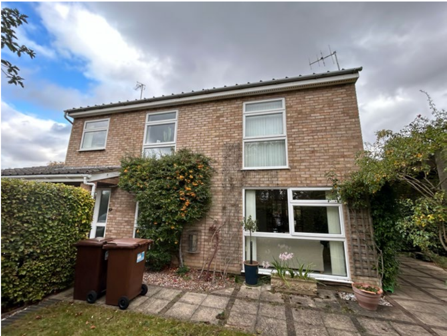
Front Facade (South-West) View from garden
