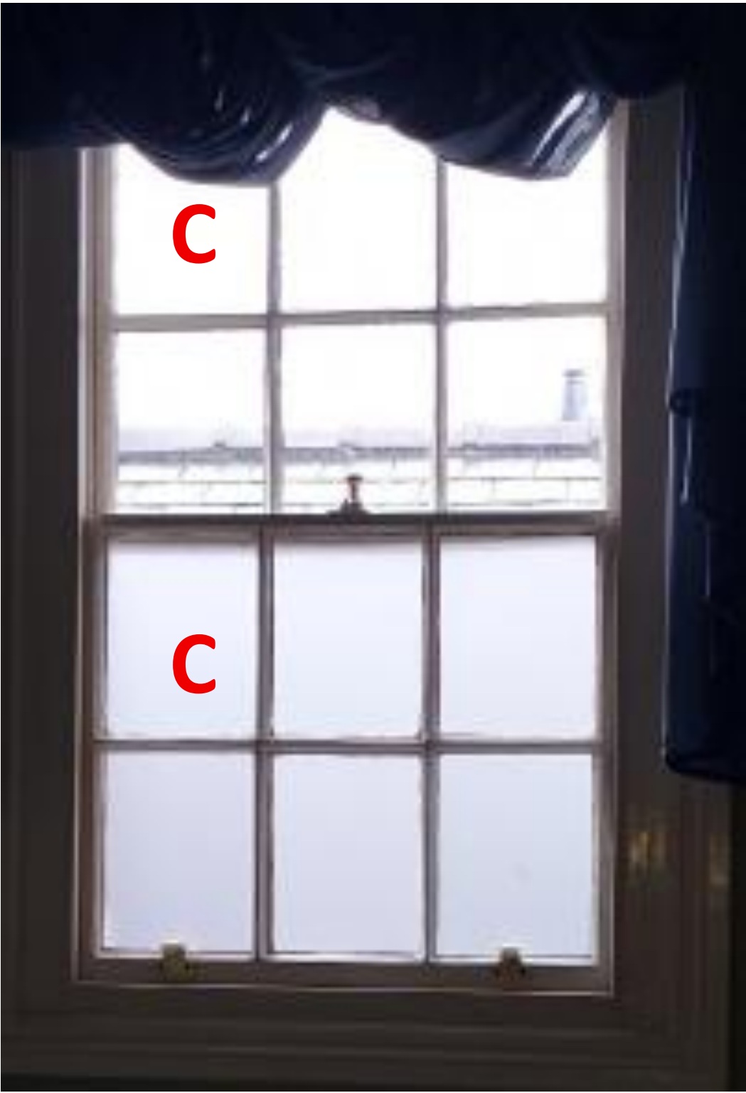
Bathroom side window 14
