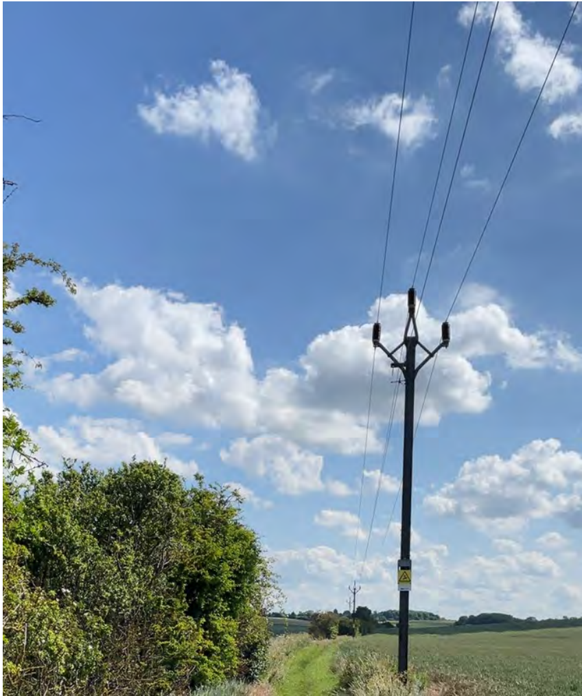
Figure 5 Overhead cables running E-W direction north of the site.
