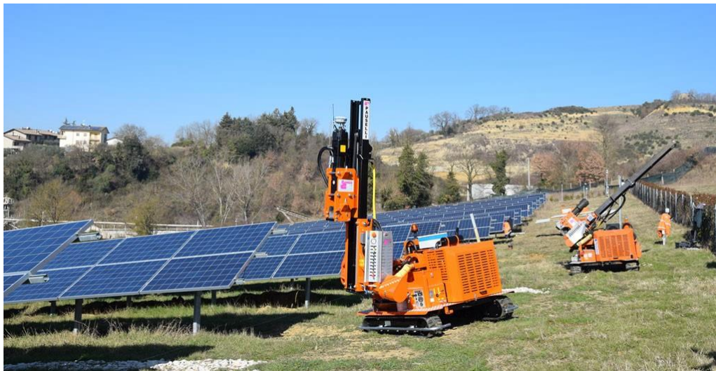
Plate 3.1: Typical GPS Solar Farm Pile Driver
