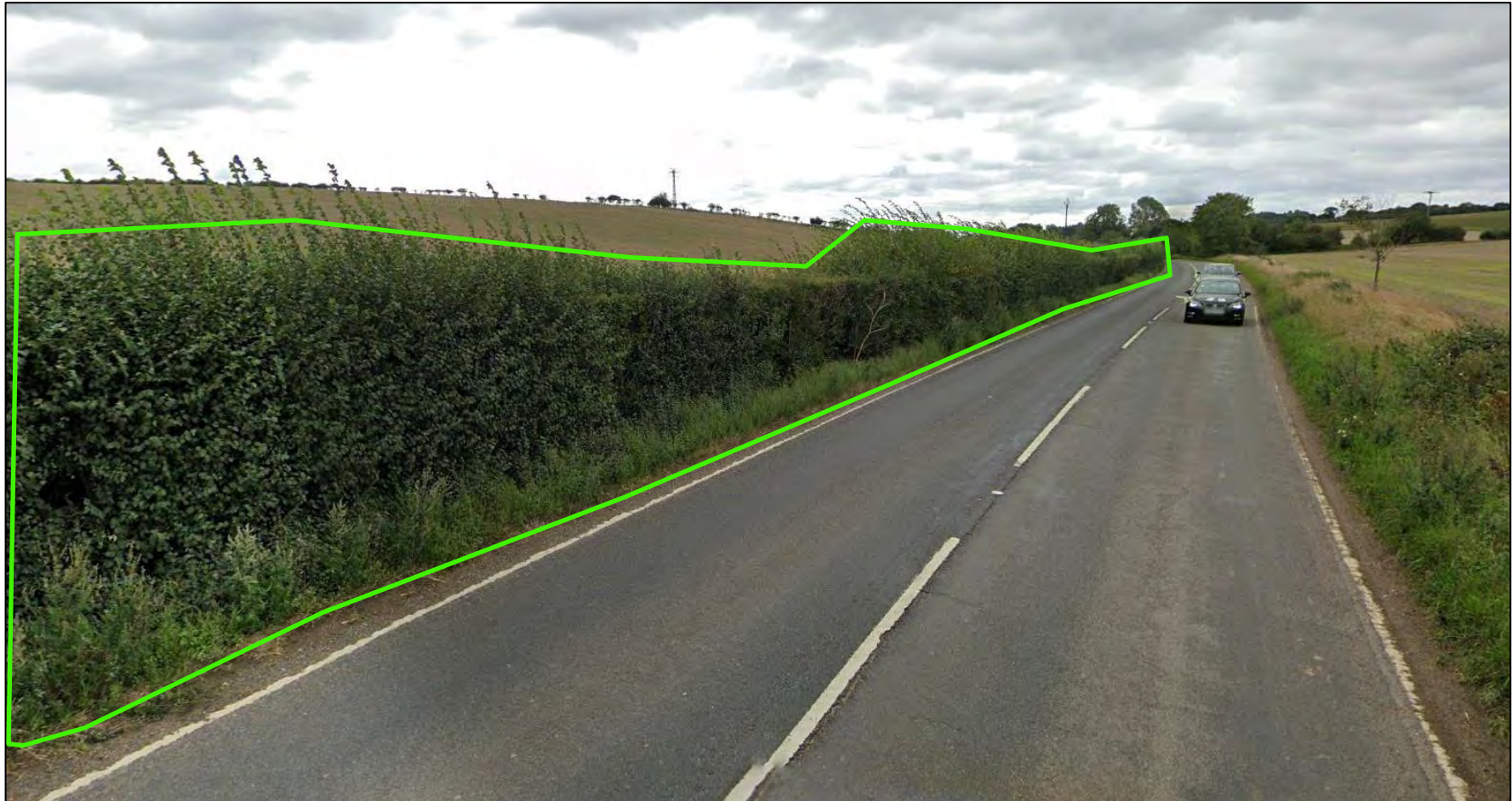
Street view showing roadside screening relevant to road receptors 48-51 (taken at road receptor 48)
