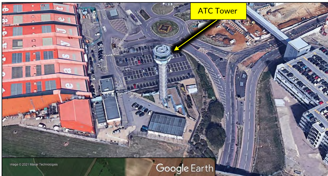
Figure 6 London Luton Airport ATC Tower
