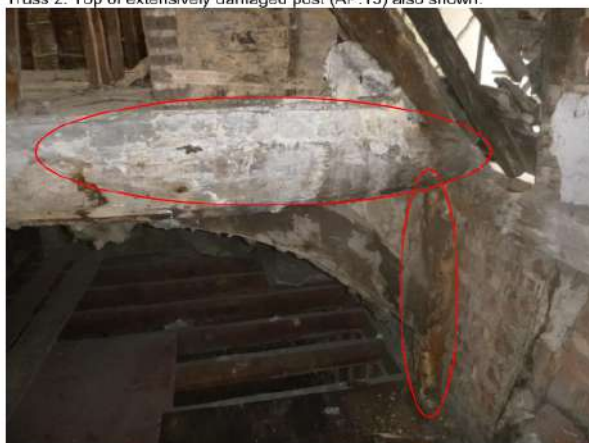
Figure 6. Extract from BM Trada survey confirming condition of existing bottom member of truss 2 (Gridline D)
