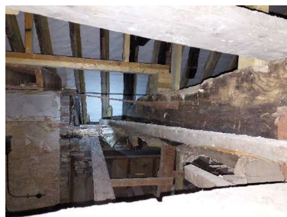
Figure 3. Photo from site visit showing vertical members and wattle and daub removed
