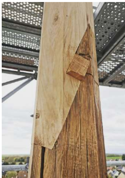
Figure 10. Example of scarf joint
