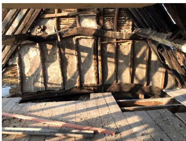
Figure 2. Existing wall prior to previous works commencing
