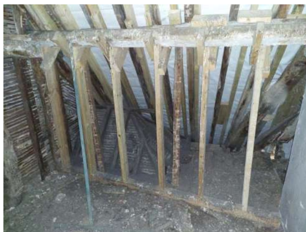
Figure 1. Purlin support and rafter strengthening as installed
