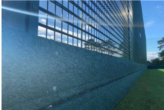
Example 0.5m containment barrier
