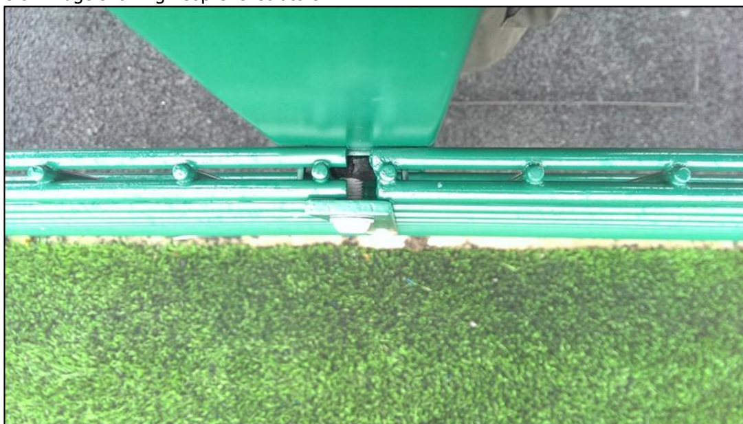
Figure 8: Image showing neoprene isolators
