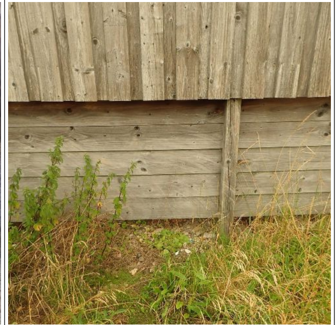
Figure 8: Building 1 - southern wall
