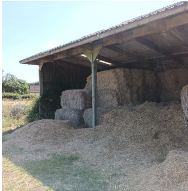
Figure 7: Building 1 - open north side
