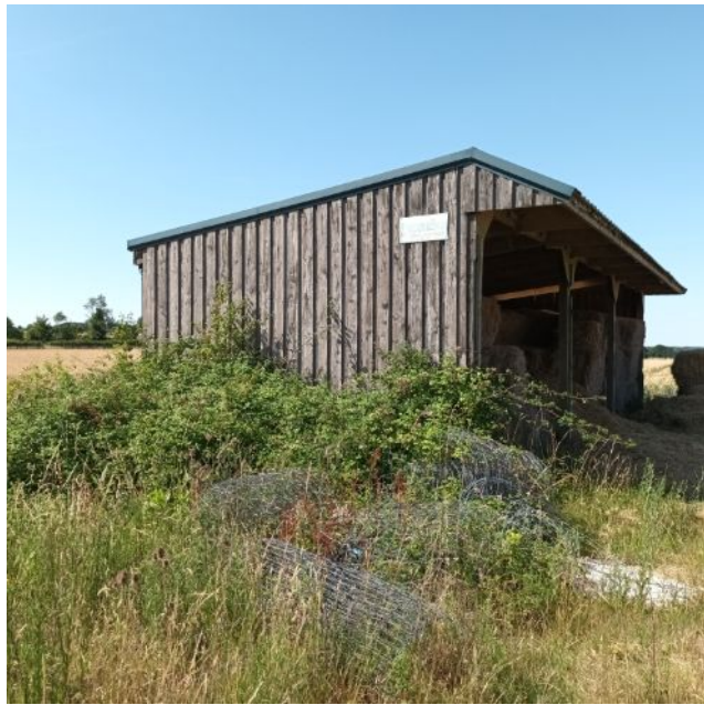
Figure 6: Building 1 [AH07] - view from east
