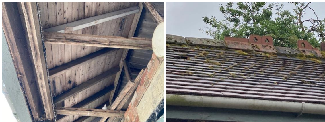
Figure 3-7 Building B Rafters in main roof and Roof showing hanging tiles
