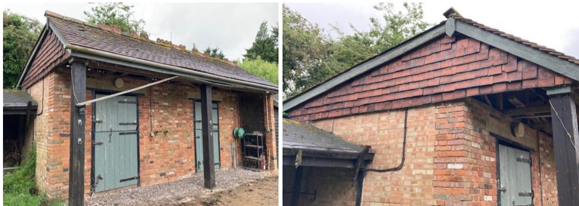
Figure 3-8 Building B-Double Stable Unit
