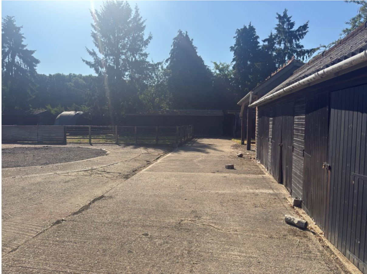
Figure 3-16 Hard standing in front of the stable buildings A-D
