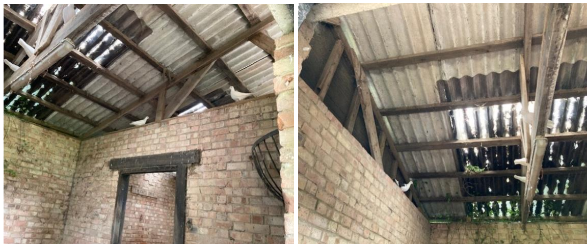
Figure 3-9 Interior of Building B
