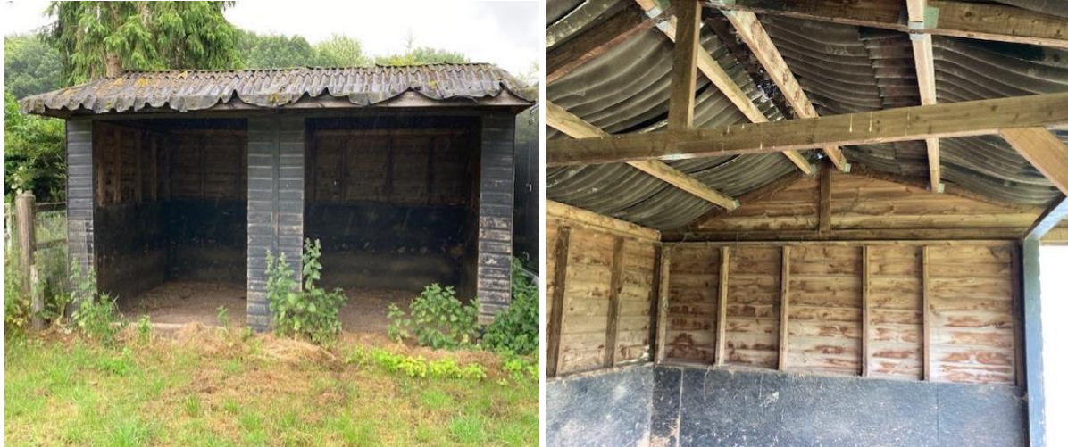
Figure 3-15 Building F Exterior and Interior
