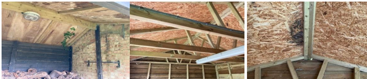
Figure 3-11 Interior of Building C
