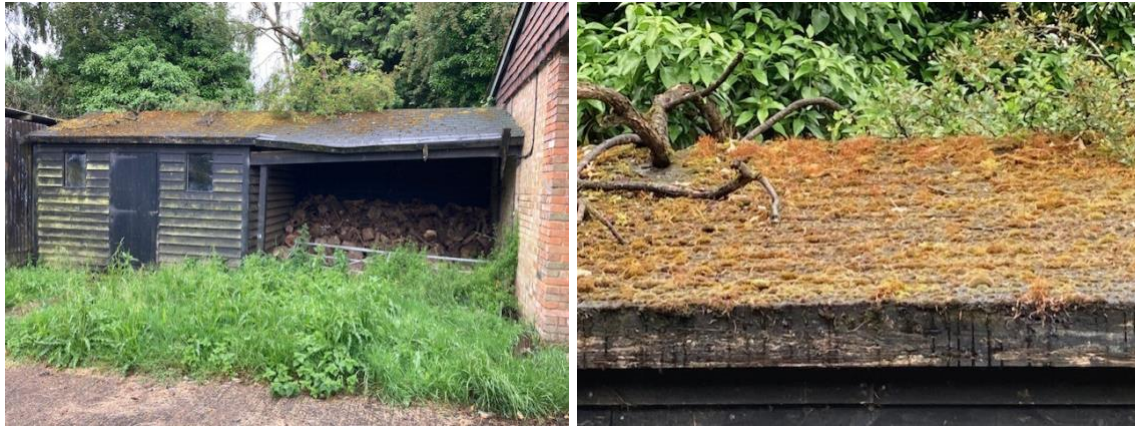
Figure 3-10 Building C- Outbuilding
