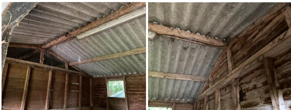
Figure 3-14 Interior of Building E
